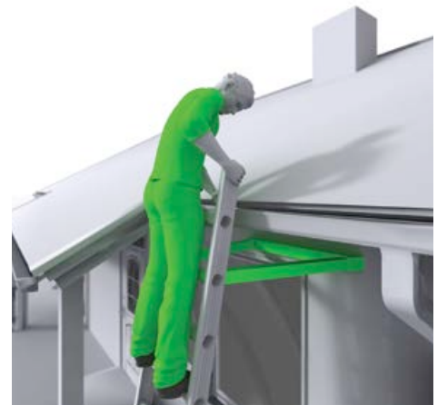
✓ Figure 4 Correct – use of a stand-off device to ensure a strong resting point. Do not rest a ladder against weak upper surfaces such as glazing or plastic gutters. Follow the manufacturer's instructions
